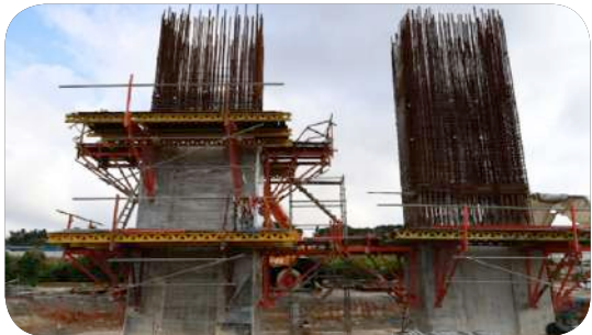
Gambar 12: Kerja-kerja konkrit berperingkat Pier 5 sedang dijalankan. Picture 12: Staged concrete works for Pier 5 are in progress.
