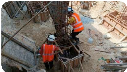
Gambar 9: Kerja-kerja membina lif dan kemudahan OKU di Stesen Batu Gajah, Perak Picture 9: Elevators and OKU facilities construction at Batu Gajah Station, Perak
