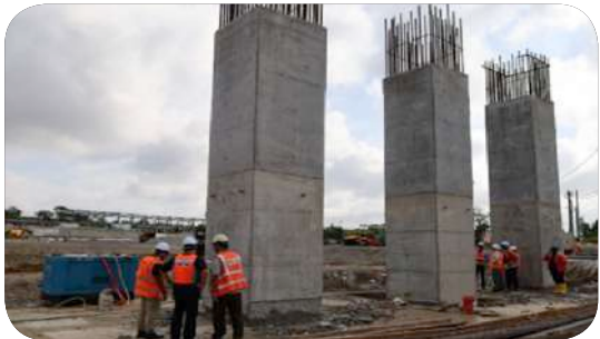
Gambar 11: Pembinaan tiang bagi Pier 4. Pasukan Projek RAC memeriksa permukaan tiang yang dibina sesudah siap kerja konkrit. Picture 11: Construction of the column for Pier 4. The RAC Project team inspects the surface of the column after the completion of concrete works.
