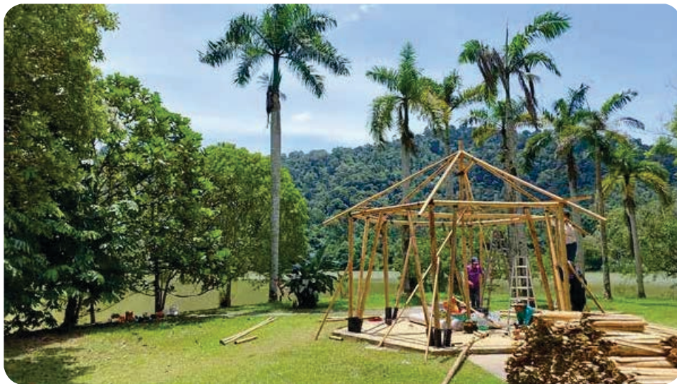
Pembinaan gazebo buluh di KBG Bamboo gazebo construction at KBG
